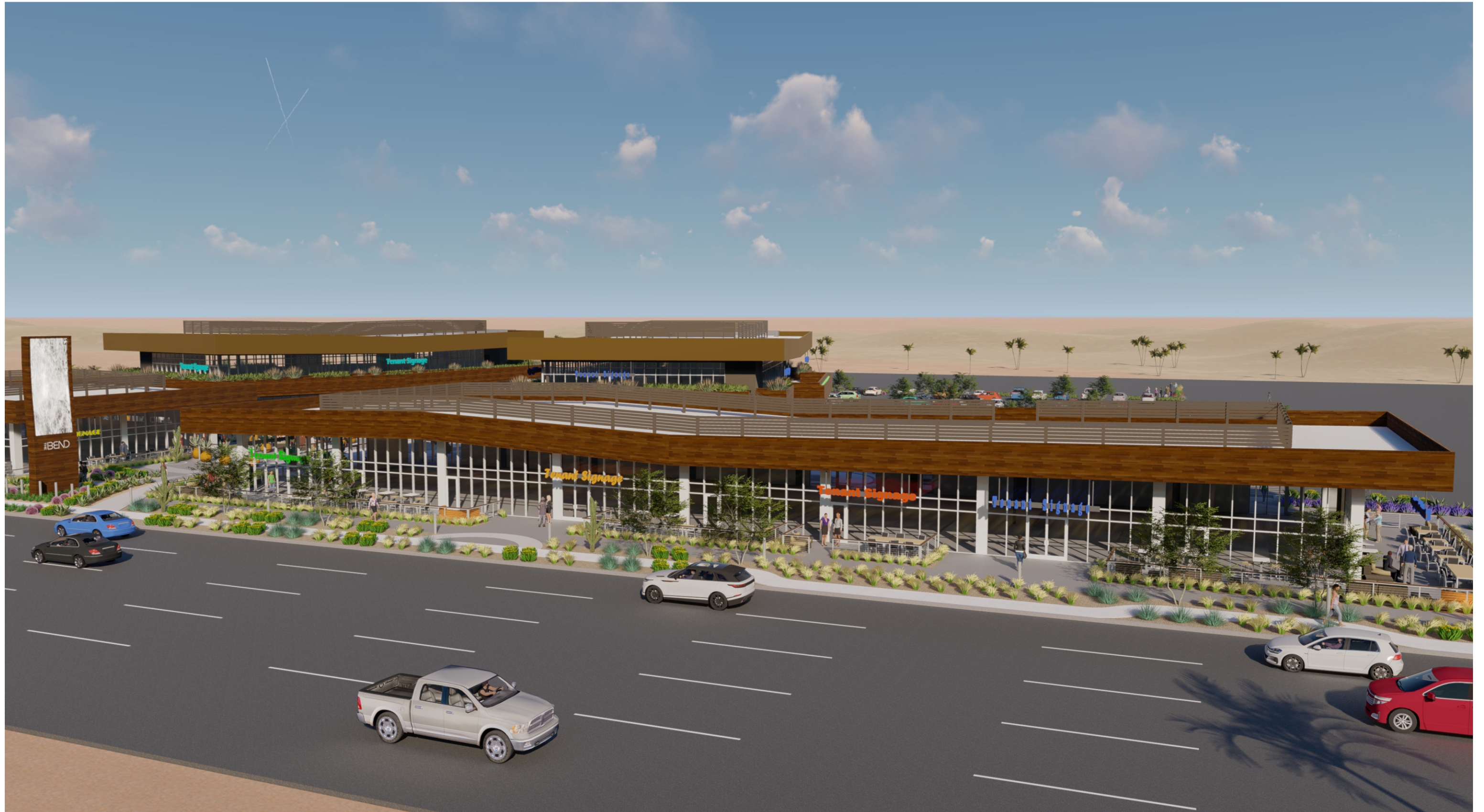
Looking Northwest at Building HILLARY
